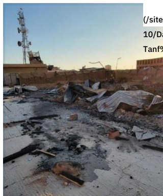
Figure 2: Damage at al-Tanf, October 20, 2021
