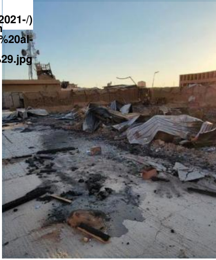
Figure 2: Damage at al-Tanf, October 20, 2021
